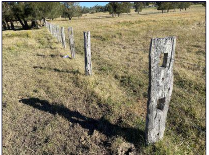
Photograph 6: Wooden fence posts along western border with evidence of former post and rail construction. View to south-west.
